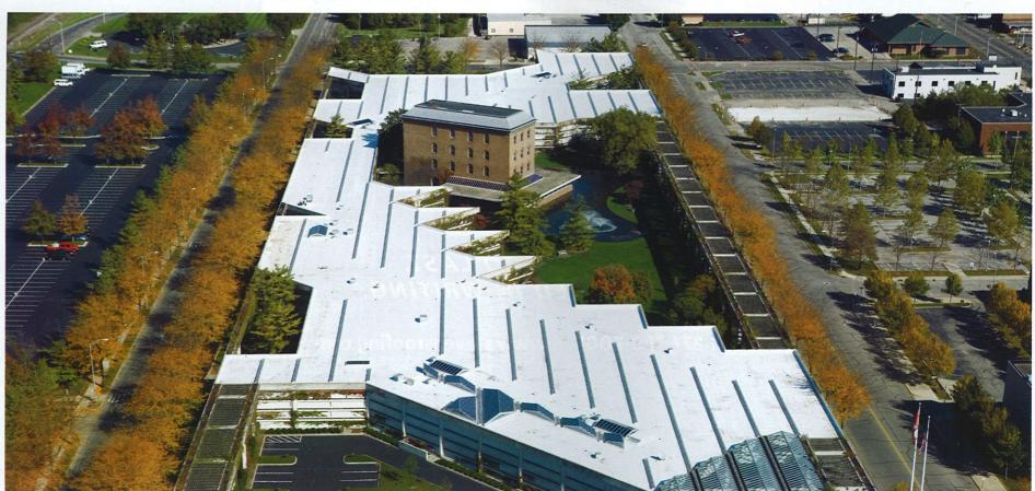
tained reflectance of 50 percent. In view of continually escalating energy costs, there is an effort underway to increase the reflectivity requirements for Energy Star qualification and to add to the standards requirements for emissivity.
