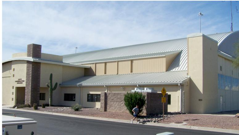
It should be noted that despite the common misconception that metal roofs are heavier roofs, the light-gauge metals used for roofing are among the lightest weight roofing materials commonly used today. In fact, only single ply systems are consistently lighter. Metal systems are appropriate not only for new construction, but for retrofitting a new roof over an existing roof, especially where roof deck designs require a lighter-weight roof covering.
