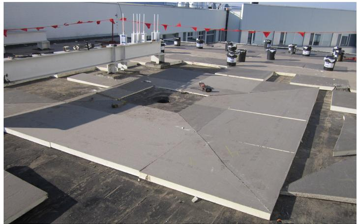
The goal of tapered roof insulation systems is to eliminate ponding/standing water on a membrane when the roof deck does not provide adequate slope. A properly designed tapered roof insulation system not only provides the necessary R-value and the support for the roof system, but it helps extend the life of the roof system because it provides the required drainage.<sup>2</sup>
