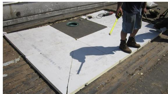
Oftentimes, building owners will agree to have a tapered insulation system installed only to have it value engineered at some point during the process, reducing the roof system’s efficiency and increasing the potential of creating problems down the road.
